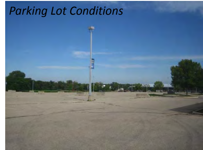
Lot Slopes to 'Back' of Campus
