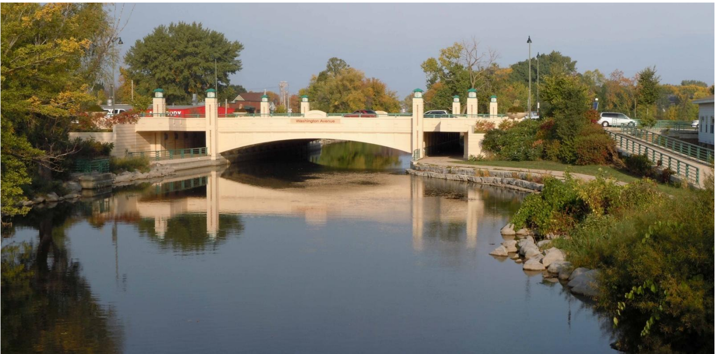
Yahara River ped/bike path at East Washington Avenue
