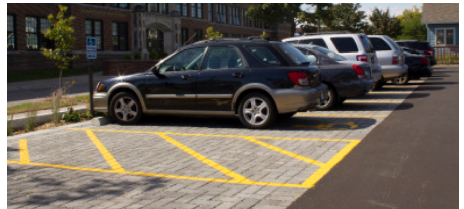
Example of pervious pavements
