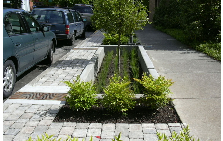
Examples of infiltration and flow-through planters
